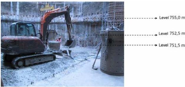
Picture 5. Removal of ground at the bottom of the shaft.
