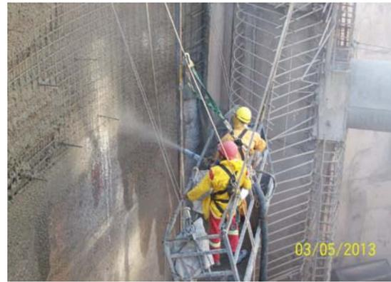
Picture 3. Reinforcement of the primary linings between levels 780 and 777.
