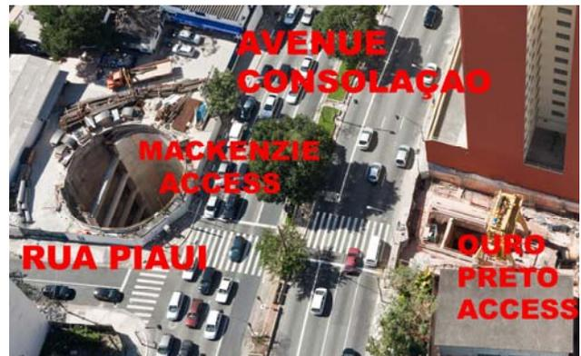
Picture 1. First shaft built in Mackenzie access.
