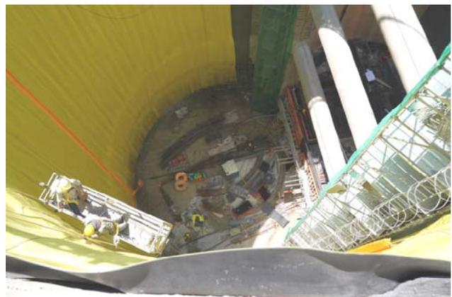
Picture 8. Waterproofing Mackenzie shaft, after finishing the primary lining.
