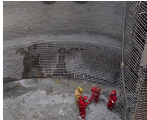
Picture 4. Reinforcement of the primary linings between levels 755 and 758.
