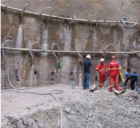
Picture 2. Drainage pipes with vacuum system.
